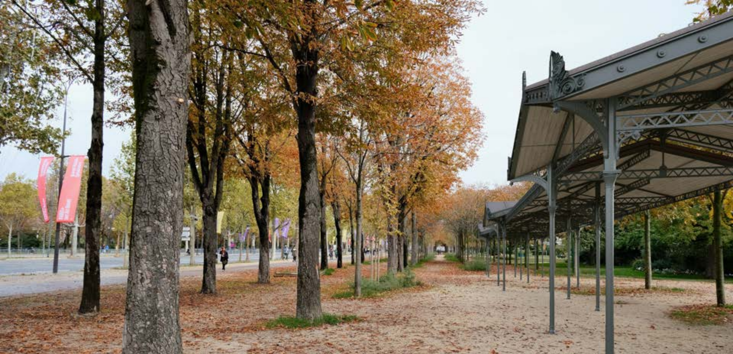
TRANSFORMING HISTORIC KIOSKS ALONG THE GARDENS
