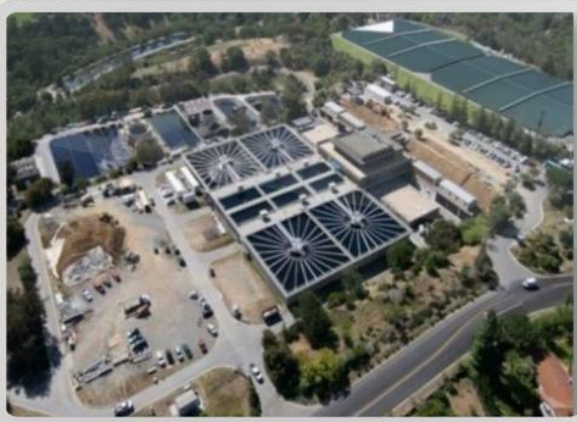
Rincónada Treatment Plant
