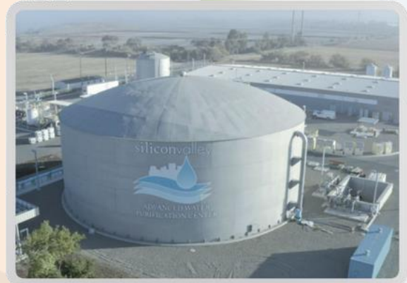
Silicon Valley Advanced Water Purification Center
