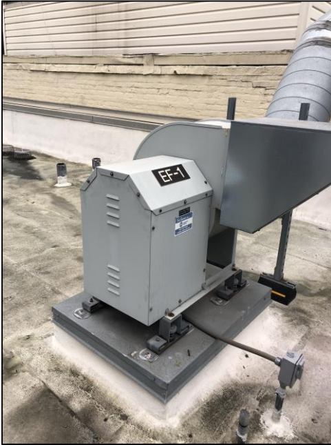
Exhaust ventilation from toilets running 24 hours/day
