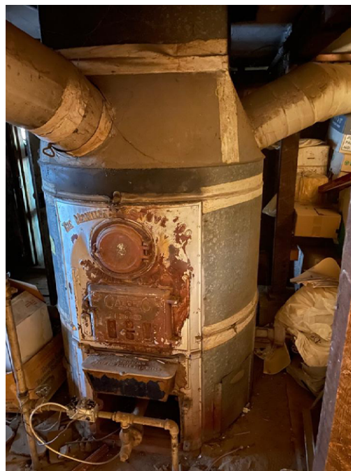
Some gas appliances far outlast their average life expectancy. This central furnace has heated a single-family home in Alameda, California, for more than 100 years.
