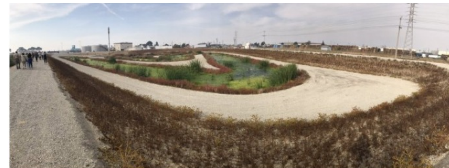
This so-called "horizontal levee" was built along the San Francisco Bay shoreline in a partnership with Oro Loma
