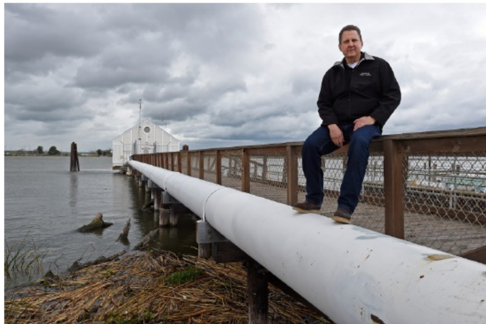
City of Antioch water treatment plant superintendent Tim Coley sits next to a large pipe that transfers water from a river pump station in Antioch, Calif., on Thursday. The pump draws water from the San Joaquin River which is then sent to a treatment plant and processed into drinking water. Antioch is one of only three cities/water agencies to receive $10,000,000 in State of California Prop 1 Grant Funding for the construction of a water desalination facility. The desalination facility will help Antioch treat water when salt levels rise in the river. (Jose Carlos Fajardo/Bay Area News Group)
