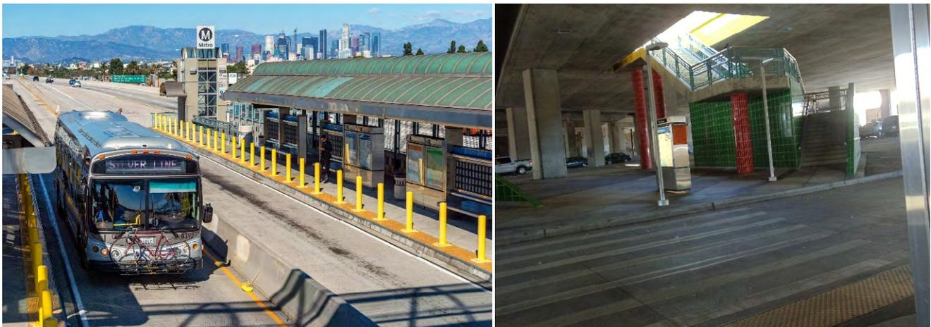
Access from above: San Diego MTS Rapid 235 line at City Heights Station, showing the freeway median station underneath the local roadway used for passenger access.
