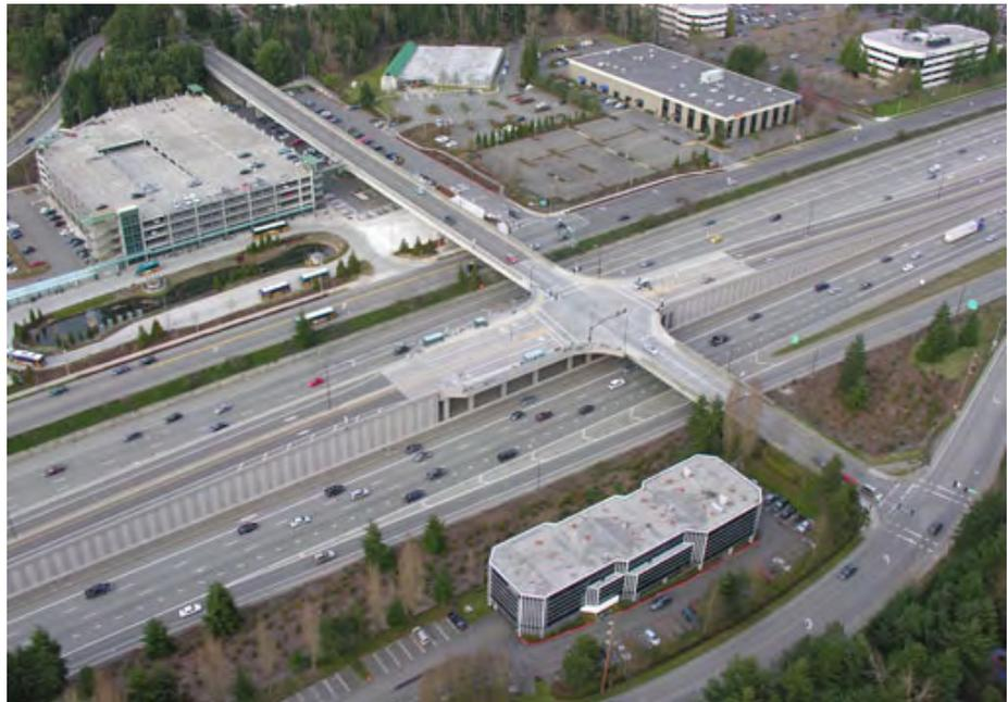
Inline stations may require less space than online stations because some portion of the total area (the station, plus the bus stopping area and potentially a separate through lane) can be located over or under the existing freeway. They do not require elevators or stairs since buses are meeting passengers at surface streets.
