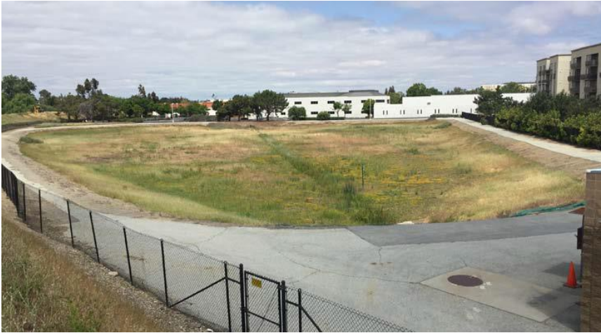
River Oaks Pump Station
