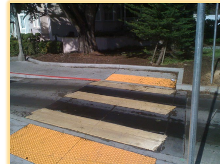
Accessible Path of Travel
