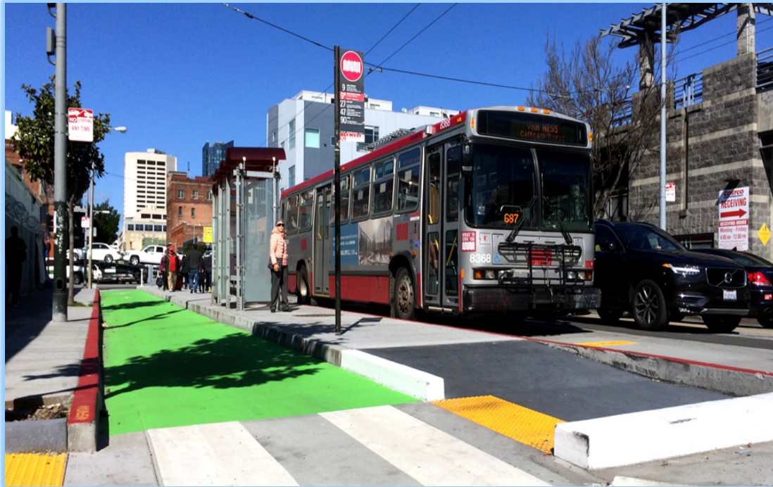
Accessible Boarding Island with a Protected Bike Lane
