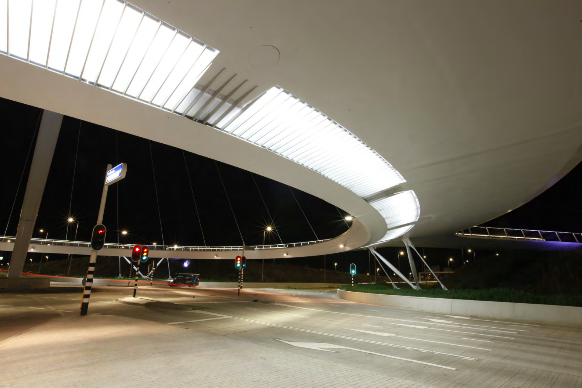
Collision Loads Concrete Barriers protect supports
