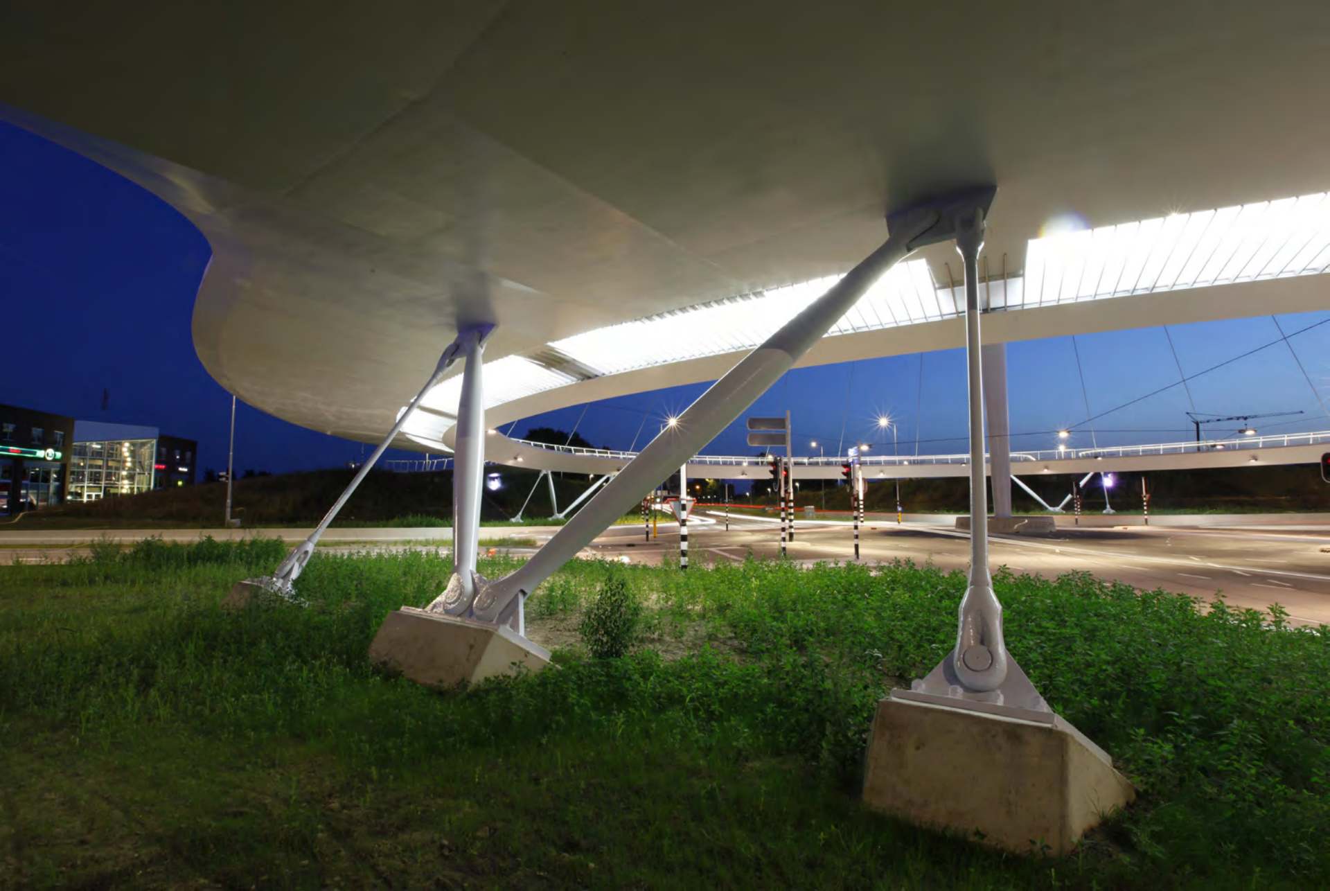
Structural Design Custom Made M-shaped supports
