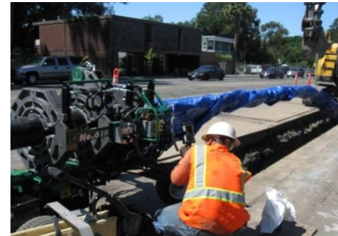
8-inch HDPE pipeline butt fusion at El Portal Drive, San Pablo
