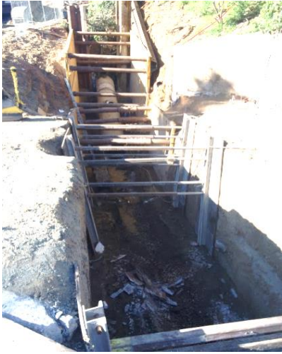
48-inch flexible expansion joint construction on 48-inch transmission pipeline at Fontaine Street, Oakland
