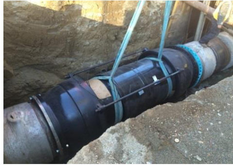
48-inch flexible expansion joint construction on 48-inch transmission pipeline at Fontaine Street, Oakland
