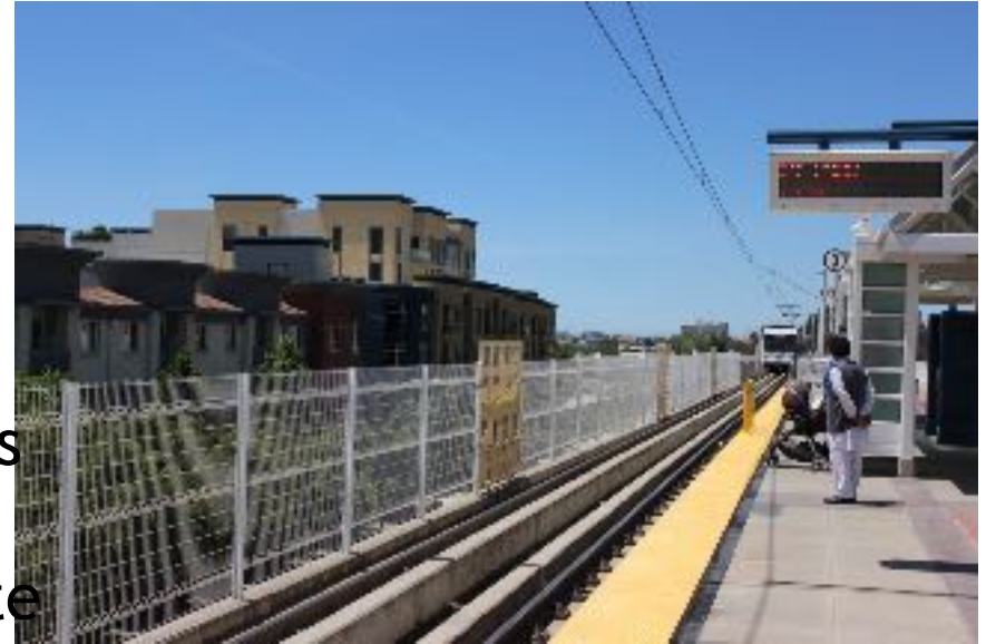
TOD located in Milpitas adjacent to VTA Light Rail line
