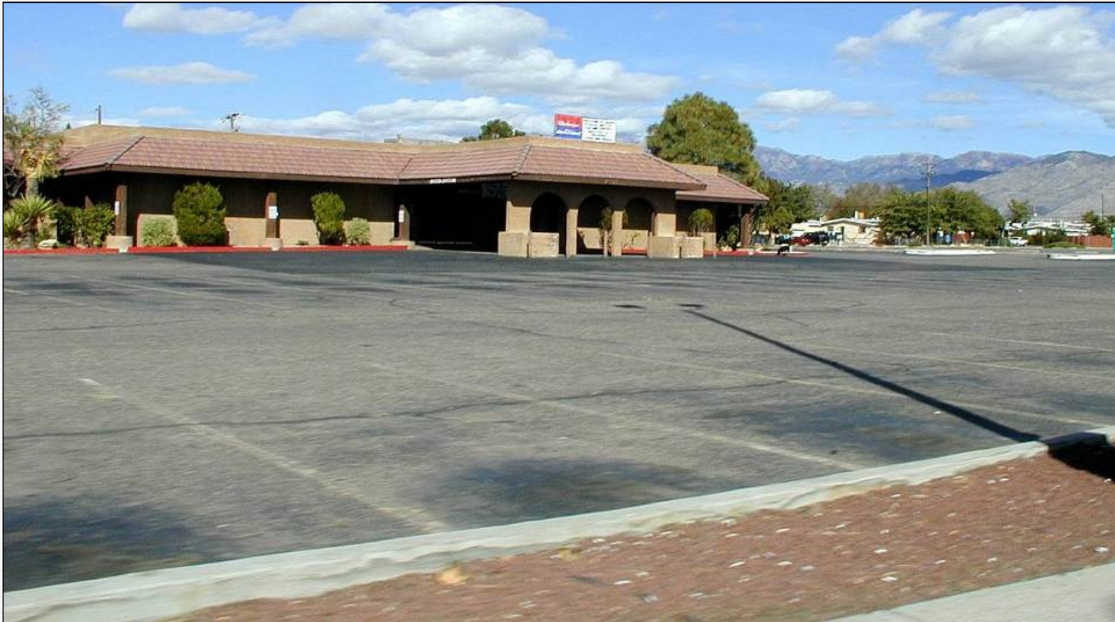
Parking between the sidewalk and buildings is not pedestrian friendly
