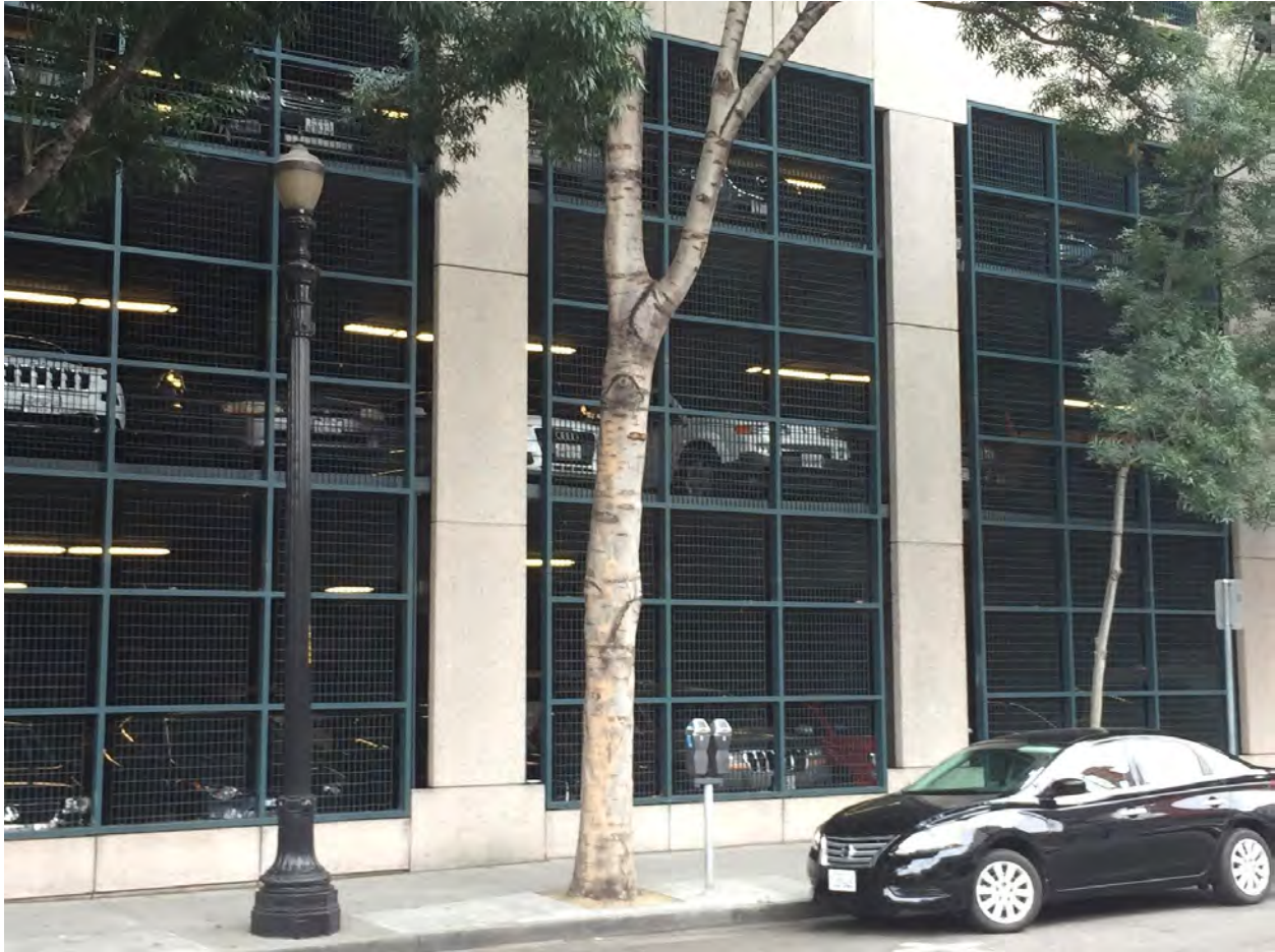
Exposed parking degrades the sidewalk environment and discourages walking. Photo by Benjamin Grant.
