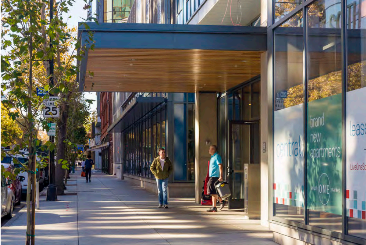
Taller ground floors provide a more pleasant atmosphere and allow for greater flexibility in the future use of the space. Photo by Sergio Ruiz.
