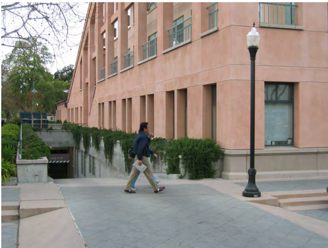
Wide garage entrances (top) feel unsafe for passing pedestrians and can discourage walking. Instead, driveways and garage entries should be as narrow as possible and should minimize disruption to sidewalks (bottom). Top photo by Sergio Ruiz. Bottom photo by Benjamin Grant.
