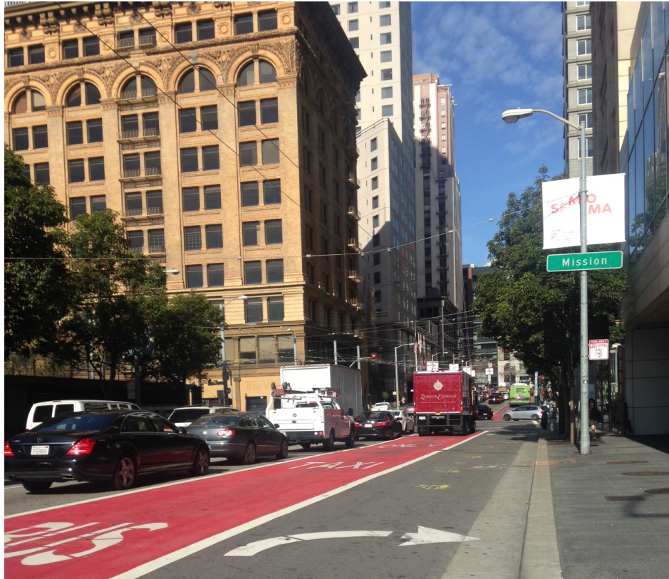
Figure 2. This image shows the right-lane bus rapid transit on 3rd Street near Mission in San Francisco. The 1- mile segment of BRT between King Street and Mission intersects with 10 curbcuts, 4 alleys, and 7 major streets. The rules and signage that manage vehicle access and flow are important ways to ensure good circulation.
