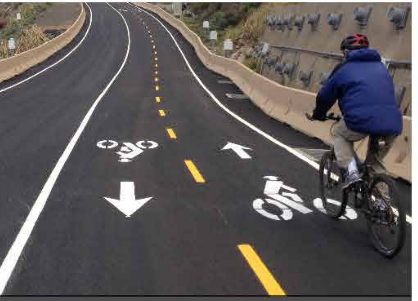
re-use of existing roadway
