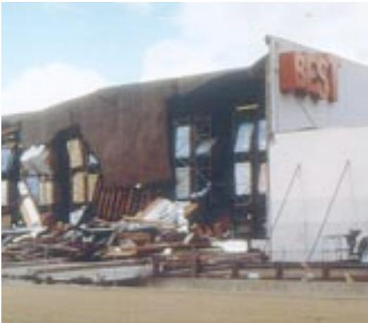
**Tilt-up.** Relatively cheap and fast to build, tilt-ups remain the structural system of choice for one-story warehouses, strip malls, and light industrial facilities. The chief deficiency in pre-1995 tilt-ups is the connection between the rigid walls and the flexible roof. When that connection fails, the concrete wall panel falls away from the building, and the roof collapses. Similar buildings with reinforced concrete block walls often have the same vulnerability.
