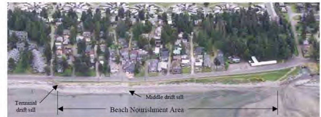
Figure 11. Oblique aerial photo mosaic of the study site, located immediately left (north) of the mouth of Terrill Creek (at right). Photos taken May 24, 2001 for WA Dept. of Ecology
