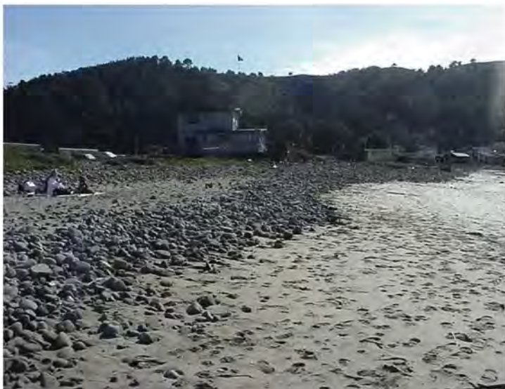
Figure 7: Picture of Cobble berms at Pacifica State Beach before the restoration project. Note the “double berm” which implies landward motion of the lower cobble berm. The house in the background was purchased by the State and demolished. San Pedro Creek mouth is on the far side of the next house, which was also demolished. Photograph © Bob Battalio, taken March 9 2002.
