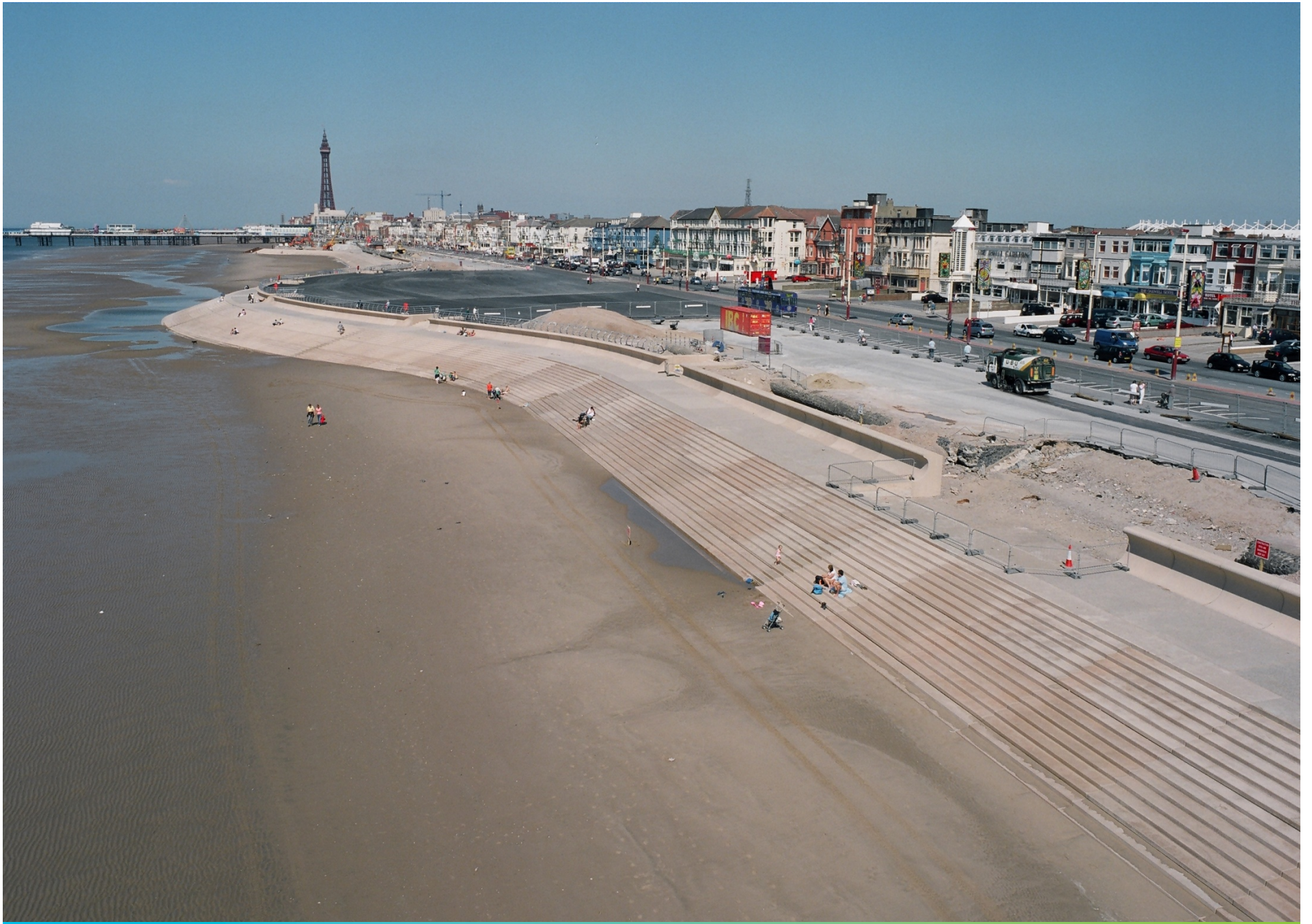
blackpool waterfront | under construction
