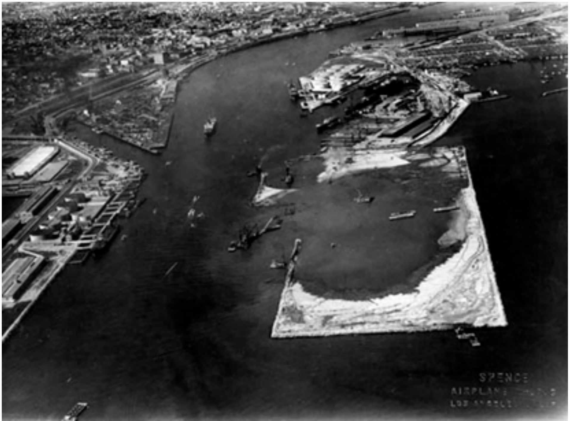
LA waterfront | building the port : filling berth, 1928
