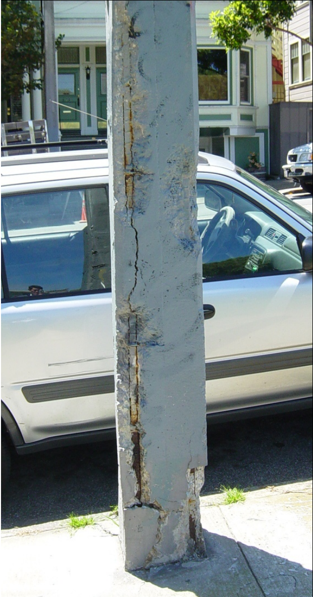
Existing Concrete Pole
