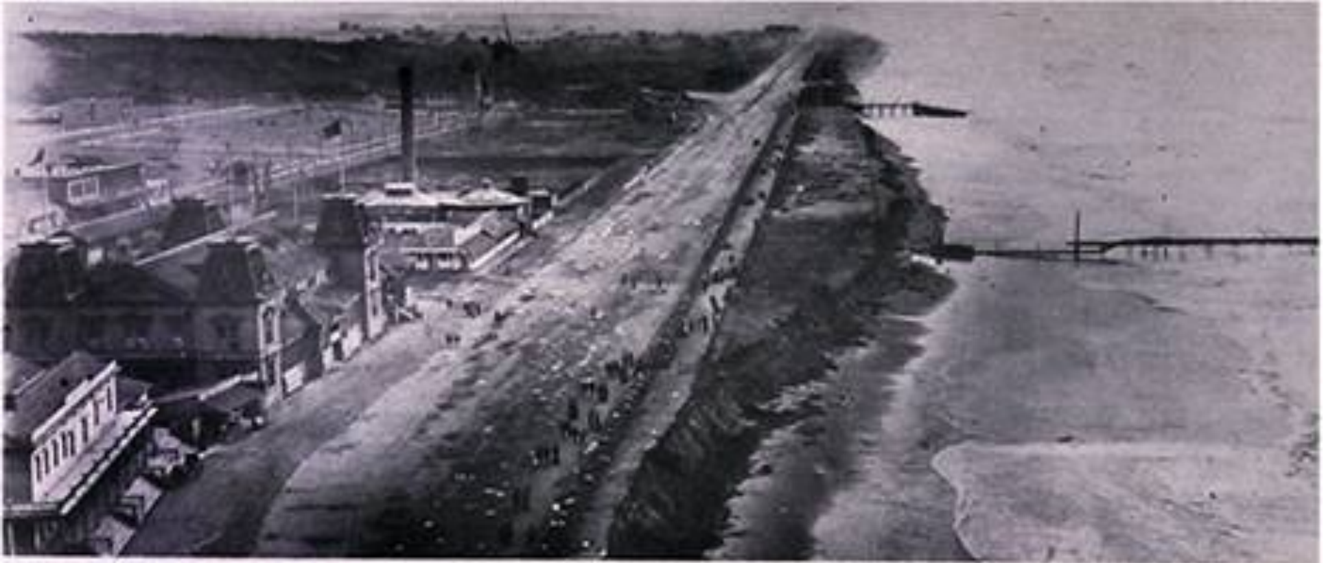
The wider the Great Highway, the more it crumbled, ca. 1907. Plenty of space for buggies and automobiles but not much beach is left. (Bancroft) The Pile Driver at Work on the first Esplanade, May 5, 1916. (Bureau of Engineers) The Cement Bleachers are in Place in Esplanade, Section A. (Calif. Historical Society)
