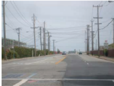
Hunters Point Blvd. at Middle Point looking east
