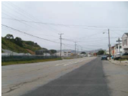
Jamestown at Griffith looking west
