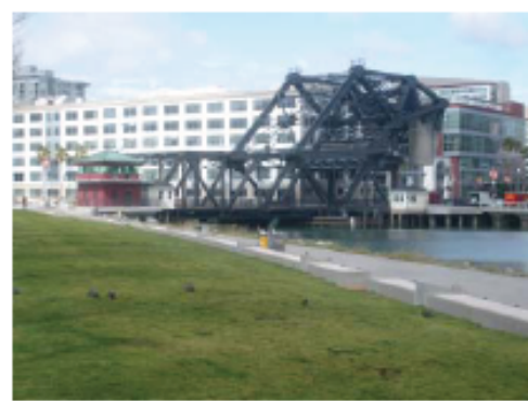
Third Street Bridge
