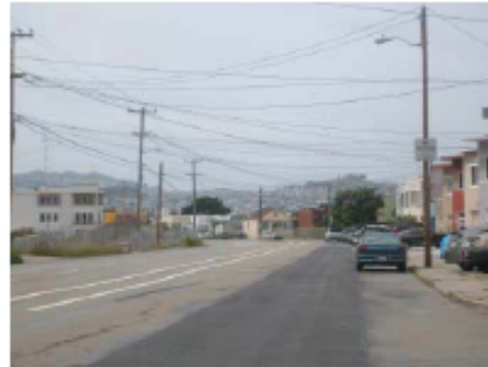
Jamestown at Griffith looking west
