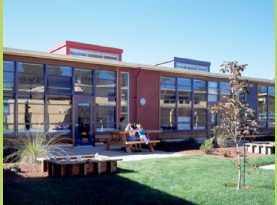
After – shear walls installed, display windows added, roof diaphragm strengthened, roof monitors added
