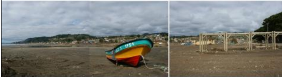
Tsunami impacted beach and campground facilities, Curanipe. Photos: Laurie Johnson
