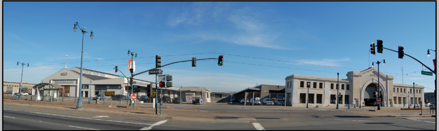
Pier 17 and Pier 15
