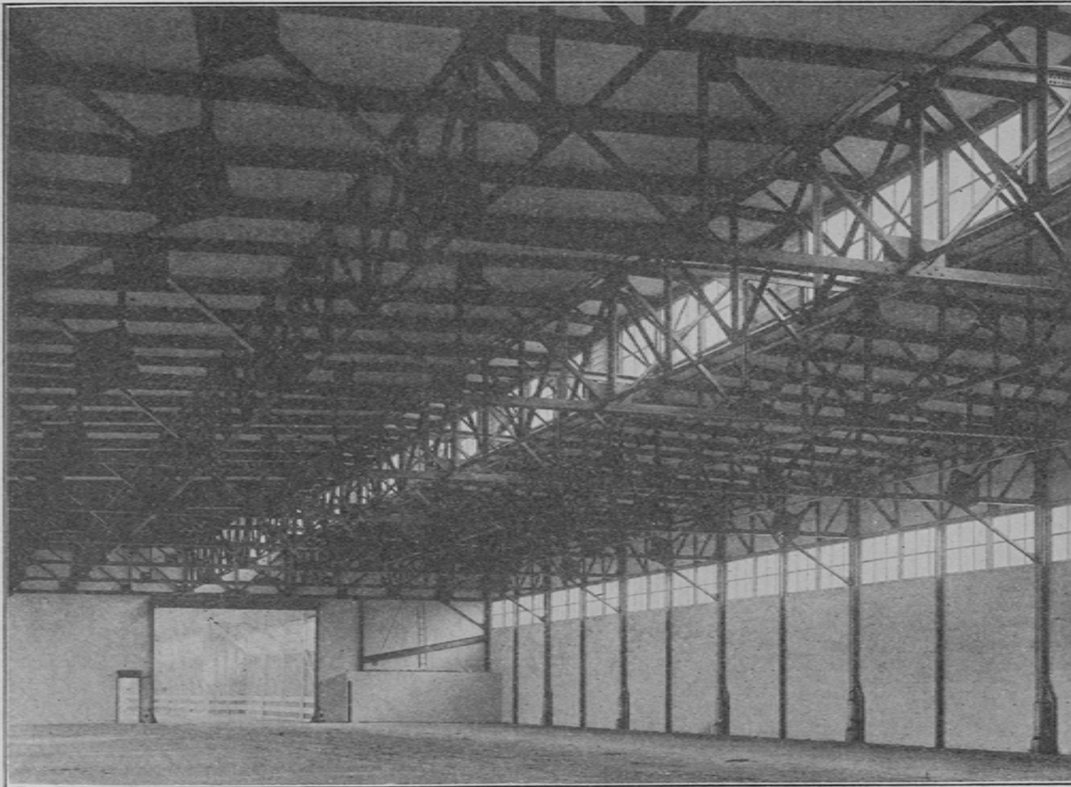
Interior of steel shed on new pier No. 36.
