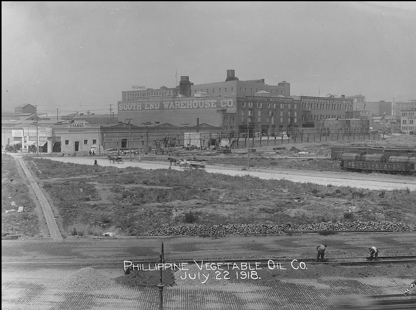
South End warehouse group Source: Port of San Francisco
