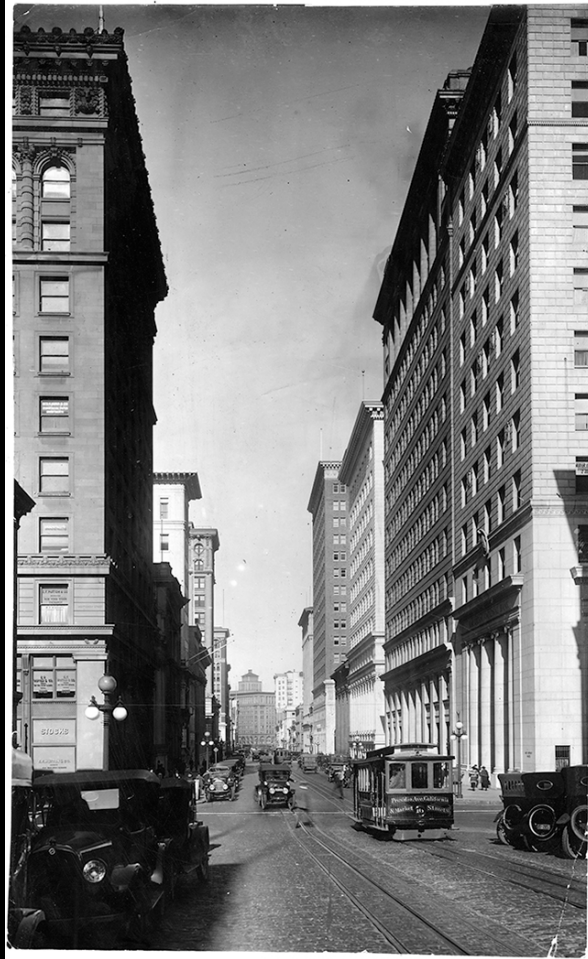
View along California Street, looking east Source: San Francisco Public Library
