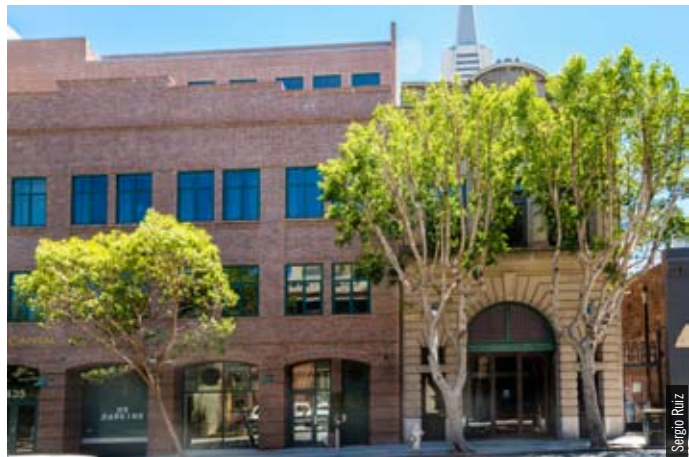
Surveys identify historic resources such as the former Engine Company No. 1 firehouse, on the right, a contributor to the Jackson Square Historic District. The building on the left, although from 1916, has been altered to the extent that it would not be considered a contributor.
