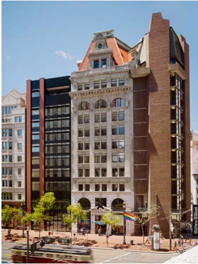
Composed of three fused-together buildings representing distinct eras, One Kearny Street is a good example of design compatibility. Through its classical composition and sensitive materials, the 2009 addition by Charles Bloszies (at left) takes cues from both the original French Renaissance Revival building (center) and the mid-century annex by Charles Moore (right).
