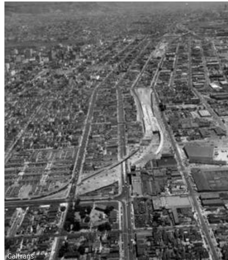
The construction of Interstate 880 during the 1950s (pictured), and later Interstate 980 in the 1980s, led to the displacement of thousands of residents and created a barrier between downtown and nearby neighborhoods.
