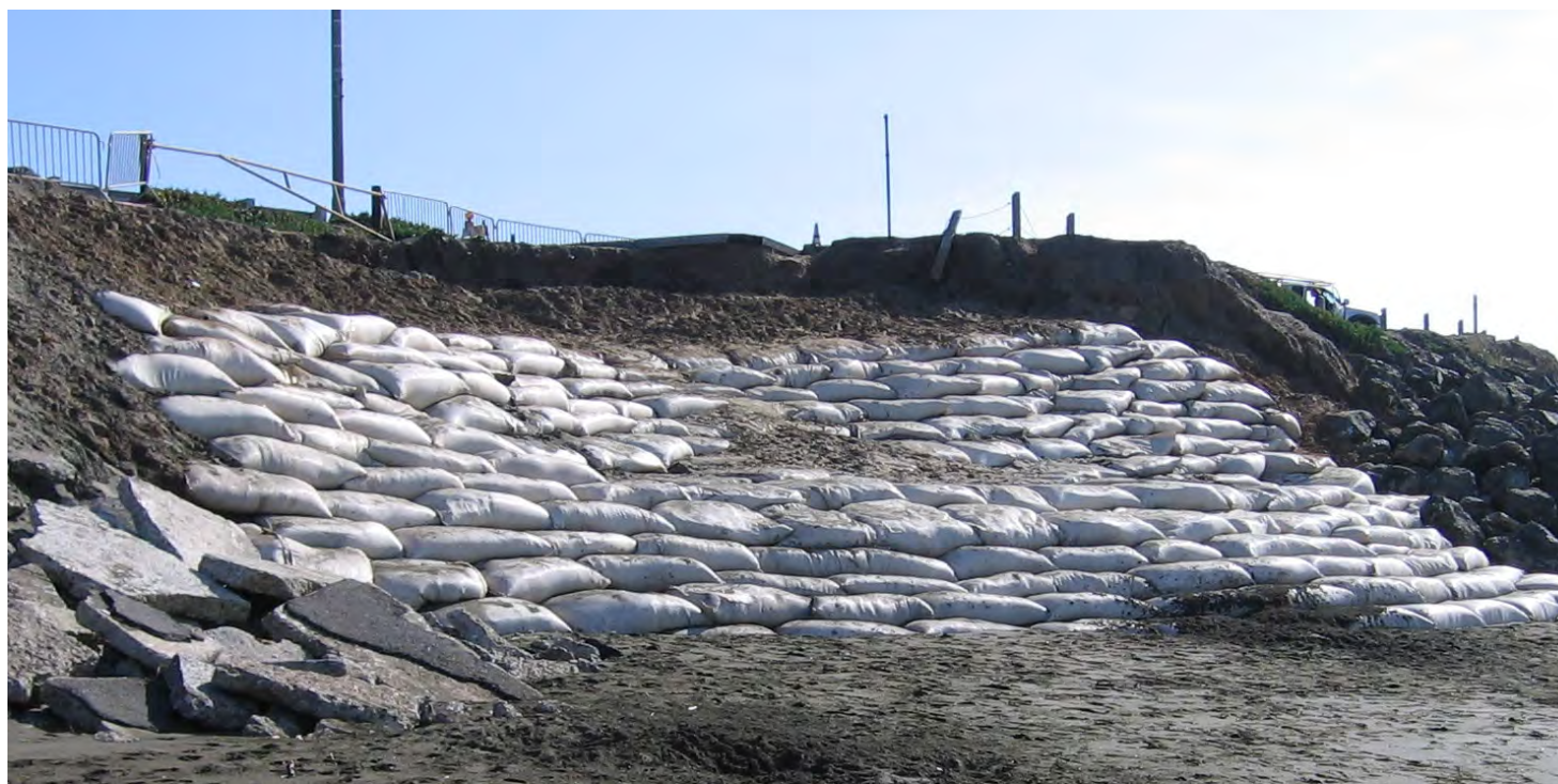
View 6 Erosion - Reach 3 (2011 Sandbag Revetment) | 2013 ESA/PWA
