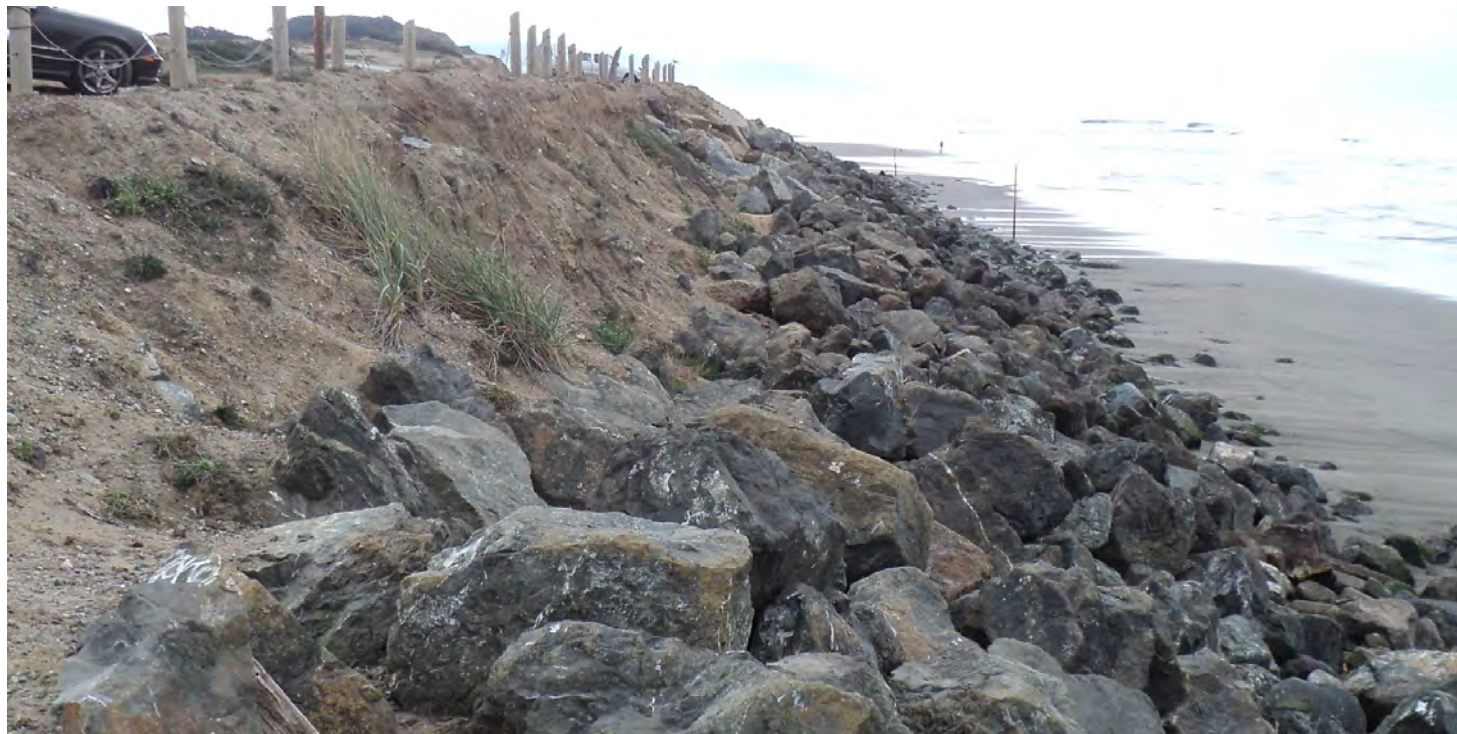
View 5 Erosion - EQR Reach (1997 Emergency Bluff Toe Protection) | 2013 ESA/PWA
