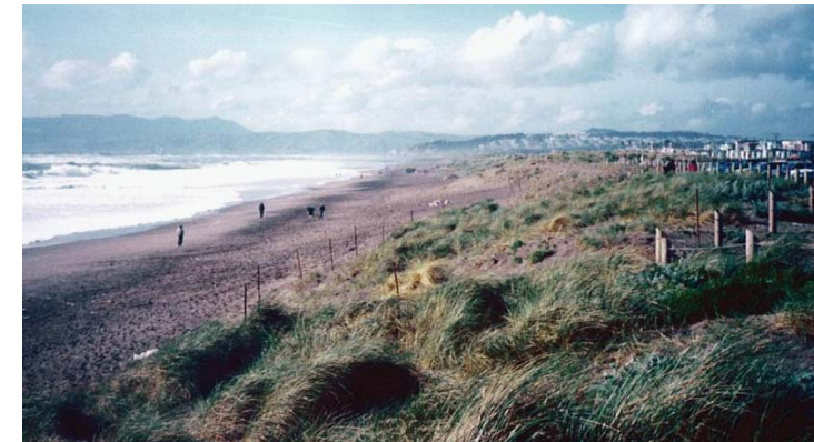
Dune restoration undertaken for the Clean Water Program
