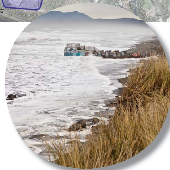
King Tide (2012), Ocean Beach's middle reach at wet-weather overflow facility
