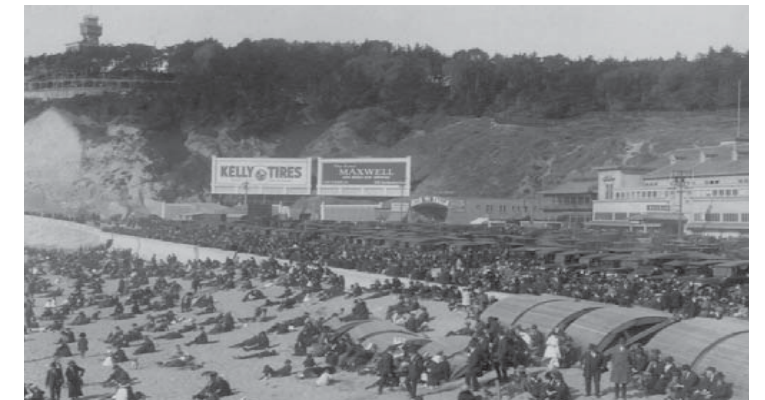
O'Shaughnessy Seawall at Kelly's Cove - (1920s to date)
