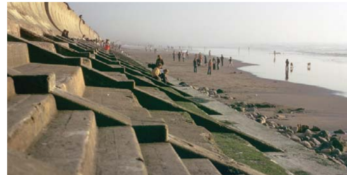
1972: The steps on the seawall are visible
