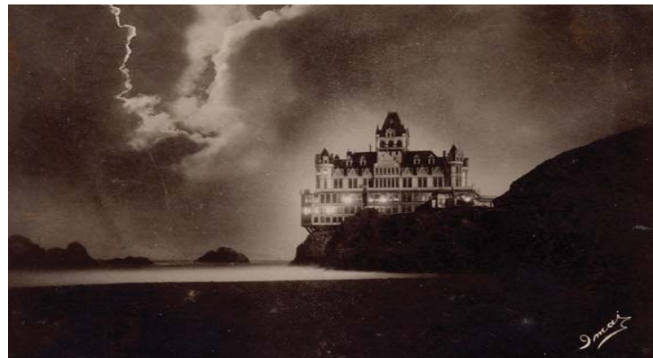
Cliff House - (1858; 1863; 1896; 1937; 2003 to date)
