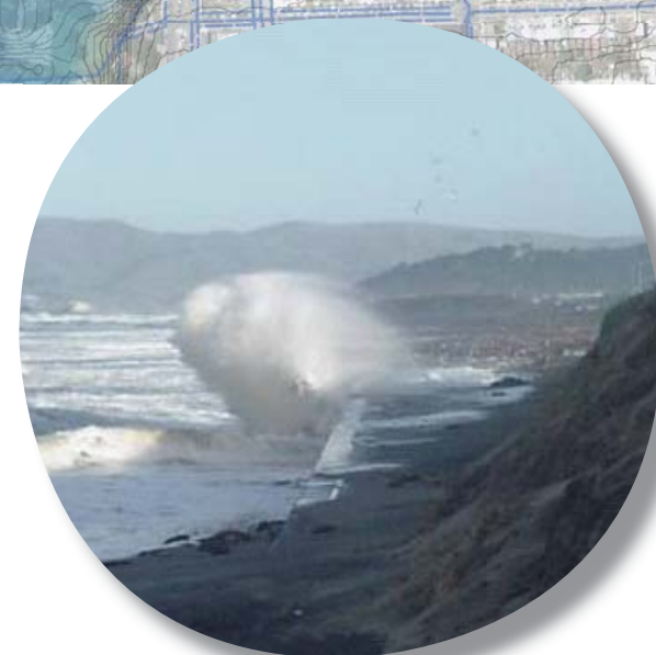
Taraval Seawall overtopping (1980s)
