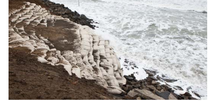
2012: Emergency/temporary repair area
