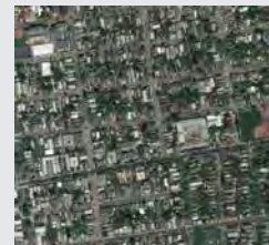
Small lot and streetcar suburbs: Medium density housing; found mostly in older San Francisco, East Bay, and Peninsula neighborhoods.
