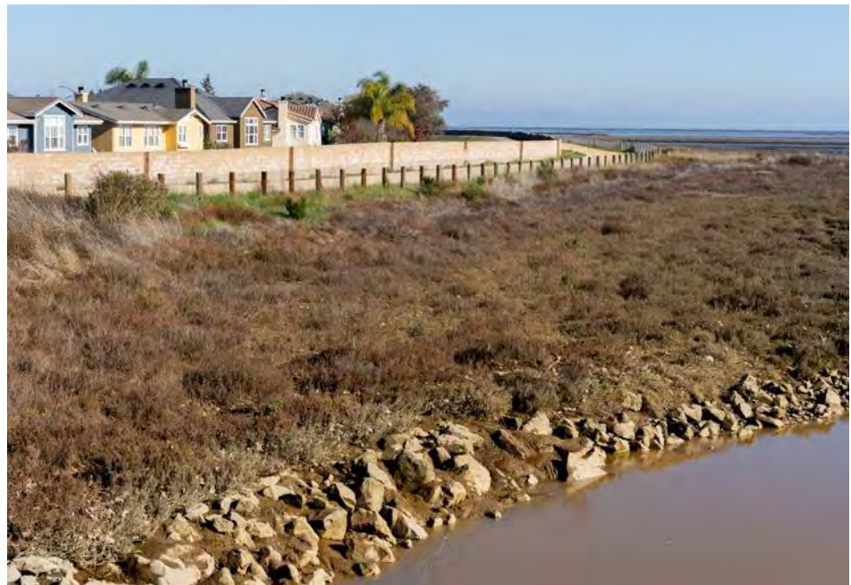
Flood wall in front of residential housing located along Hamilton Wetlands in Novato (Photo by Shira Bezalel, SFEI)
