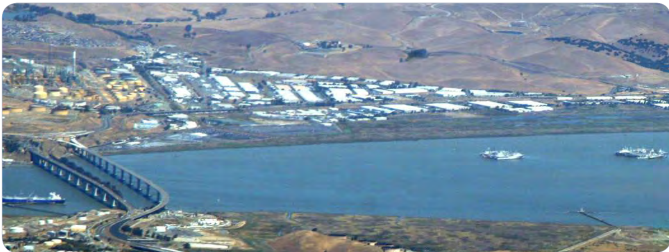
View looking north of the Benicia-Martinez Bridge in the Carquinez Strait, showing heavy industry fronted by marsh in the Carquinez North OLU (Photo by Doc Searls, CC BY-SA 2.0)
