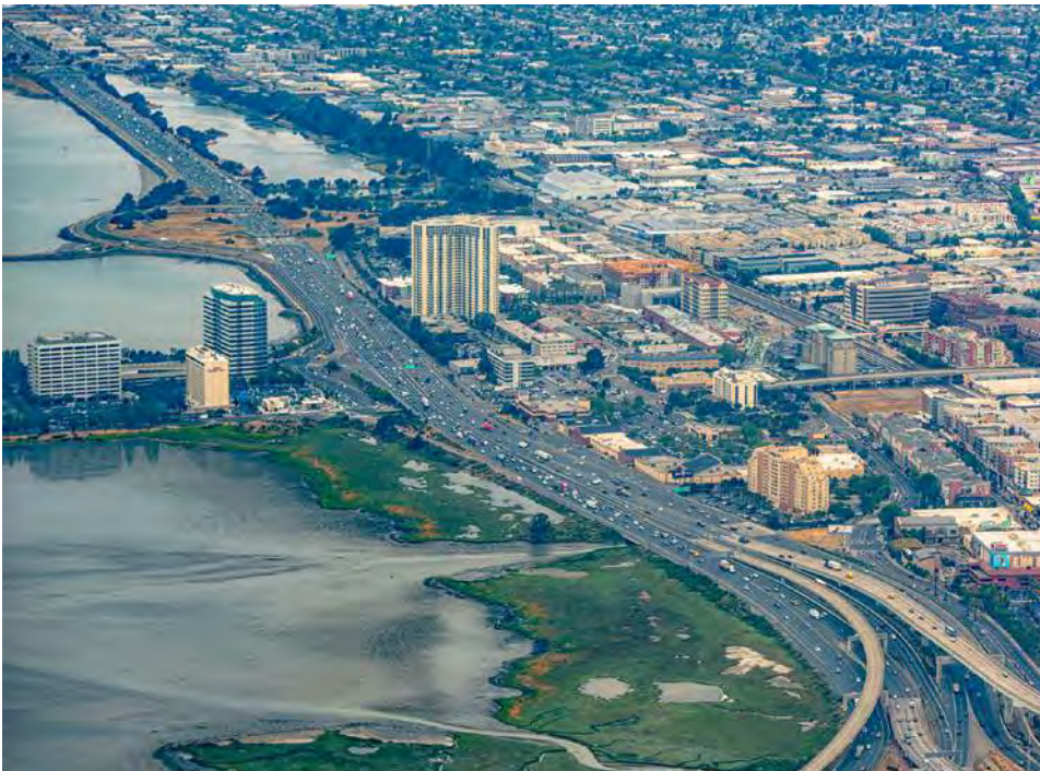
East Bay Crescent OLU (Type G) has little accommodation space along its shoreline due to extensive development and transportation infrastructure built on top of historical baylands; however, some marsh and shallow areas exist, allowing for more nature-based adaptation options compared to Type D (Photo by Jay Huang Photography, CC BY 2.0)
