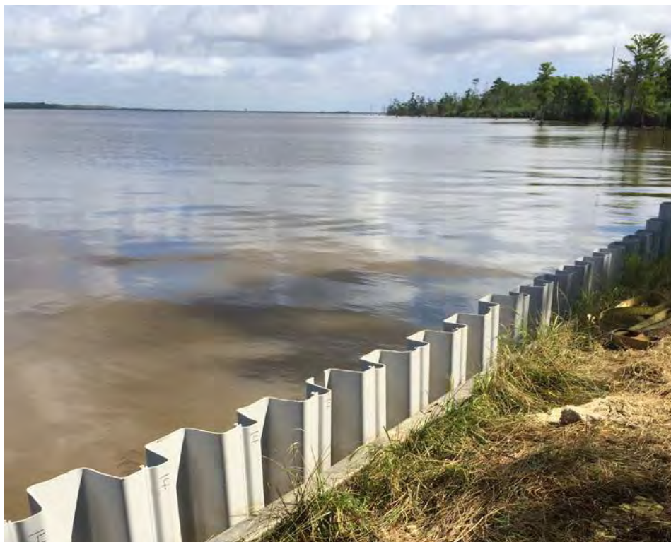
Bulkhead along the North Carolina coast (Photo courtesy USFWS)
