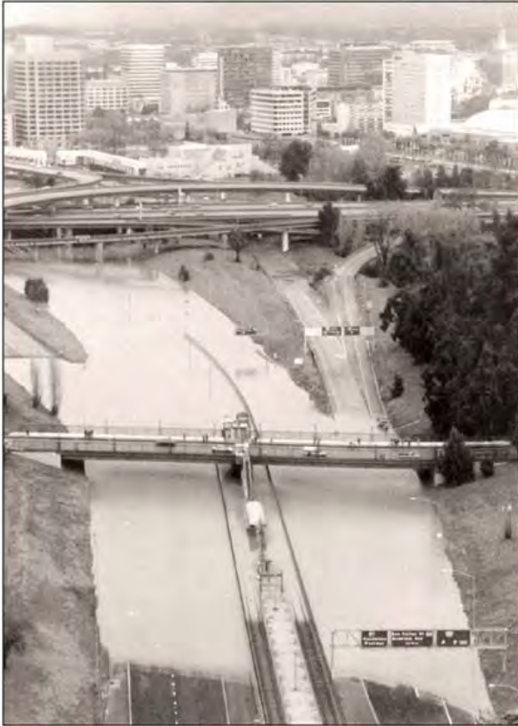
Floodwaters spill onto Highway 87 in downtown San Jose during the flood of 1995. Image courtesy Santa Clara Valley Water District.
